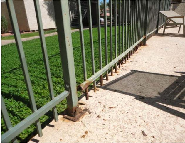
The pool area wrought iron is in poor condition and should be replaced at this time. This wrought iron is continuously hit by sprinkler water.
