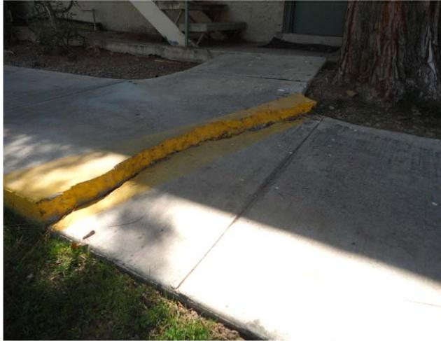
There are several areas throughout the property where the concrete sidewalks are unsafe. Since there doesn't appear to be a line item included in the operating budget for concrete repairs, this component includes a provision every five years to begin addressing concrete repair/replacement issues.
