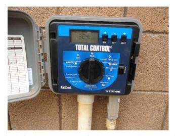
This component will accumulate funds for the replacement of irrigation controllers as needed. We located one controller, an Irritrol, Total Control 18 station in Tract C.
