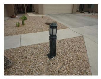
These are decorative, metal bollard light fixtures that line the streets. This component budgets to convert these fixtures to LED per the proposal provided by JFK Electrical Contractors for \$2,098.
