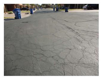
This component includes a provision to pulverize the existing asphalt, removing excess materials, grade and compact pulverized material, and repave with 2.5" of new asphalt.
