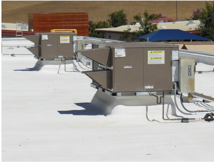
Figure 2 – Typical result of an approved method of a new Air conditioning unit's installation using an 8-inch mounting curb
