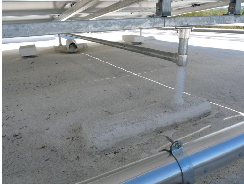
Figure 3 – Typical solar panel installation with approved 8 inch spacing between the lowest part of the solar frame material and the roof elevation
