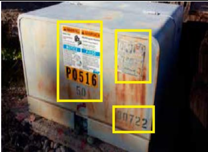
Exhibit 3. SRP Pad Mounted-Equipment. Owners must NOT paint over stenciled numbers, reflective stickers, or instructional/ warning decals, as shown in the highlighted areas on the image above.
