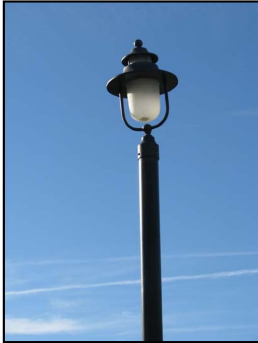
Pool Area Pole Lighting
