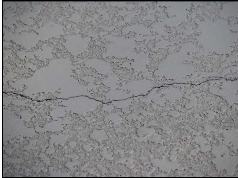
Kool-deck Cracking
