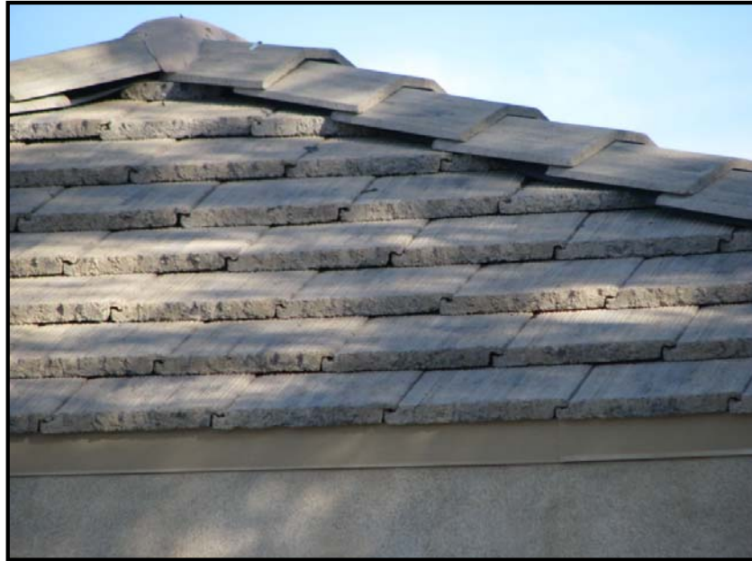
Ramada Tile Roofing
