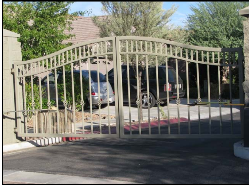
Vehicle Entry Gates
