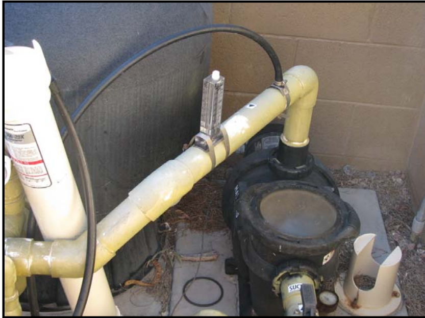
Pool Pump & Motor
