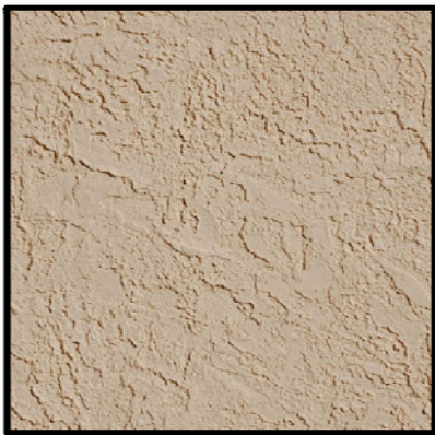
Existing Stucco Texture Good Condition
