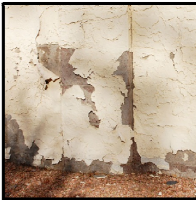
Property Line Fence In Need of Repair
