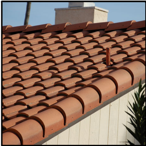
Existing Roof Tiles
