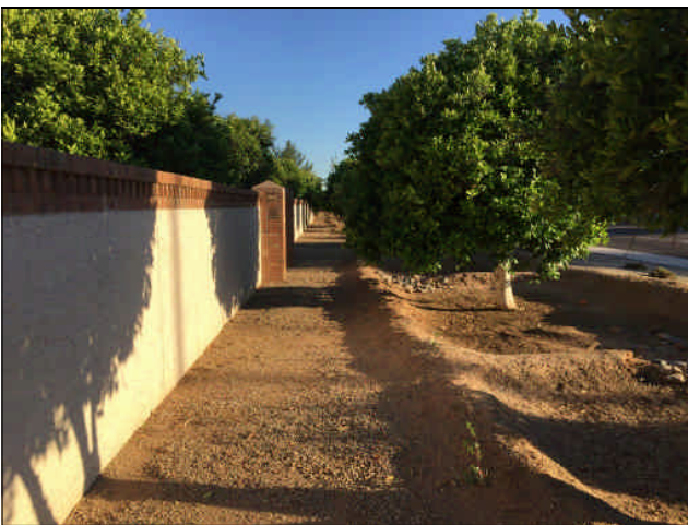
Stucco Wall Paint and Repair
