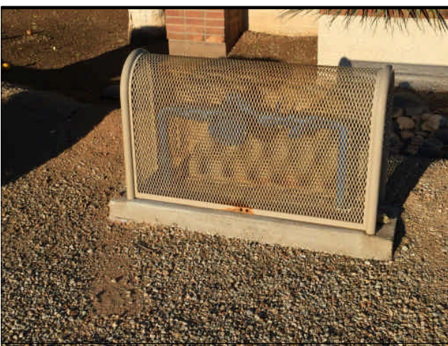
Backflow Preventer Replace
