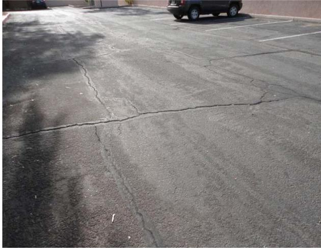
The asphalt was crack sealed, repaired, seal coated & restriped in mid-2016. We don't recommend doing any more asphalt maintenance prior to the rehabilitation project scheduled to occur in 2022, unless repairs are absolutely necessary due to safety concerns.
