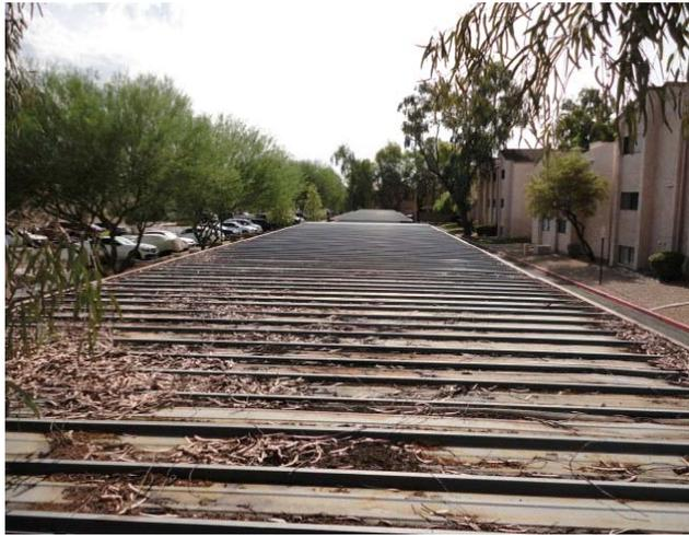
We are not budgeting to replace the corrugated metal carport roofs because they should last indefinitely. However, the condition of these roofs should be monitored over time, and if future replacements are anticipated, we will include a provision for such in a future update of this report. Should the client wish to budget for these roofs at this time, we will revise this report to include these roofs at their request. Minor repairs should be handled on an “as needed” basis using operating funds.
