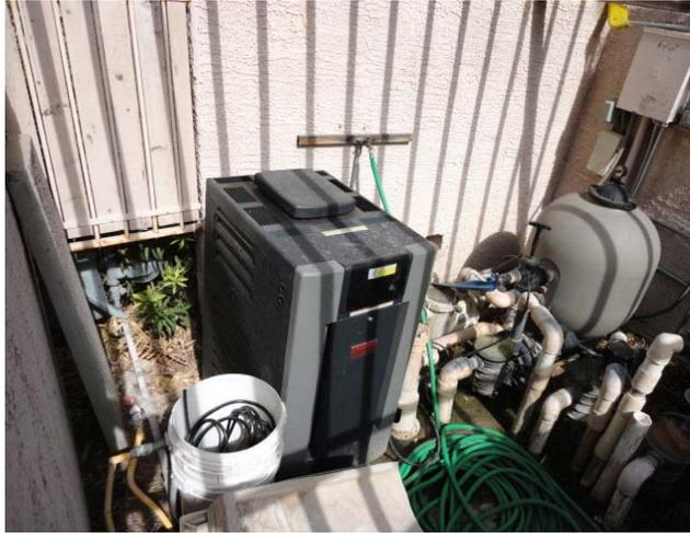
This is a RayPak, 199,000 BTU input heater that was installed in late 2017 at a cost of \$2,600.
