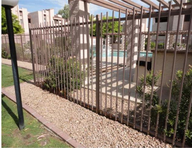
The age of the wrought iron fencing & gates at the pool area is unknown. However, it does not appear to be the original fencing. For budgeting purposes we have used 2004 as the basis for aging it. The pool fencing is severely rusted in multiple locations, and unsteady in a couple locations. This component includes a provision to replace the following pool area wrought iron on a 20 year cycle.
