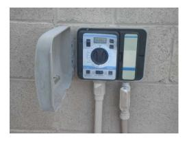
New condition. Irritrol 6-station irrigation controllers, model RD-600. Will be replaced in 2019 at the same time as irrigation and landscape improvements are performed.
