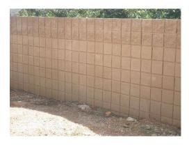
Poor condition. Faded and cracking from trees and irrigation. Recommend painting soon. Last painted in 2008 for \$13,697. Some block walls under the view fence in hard to access areas due to terrain and vegetation. Masonry walls painting to coincide with metal painting see asset ID 1006.
