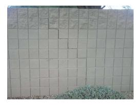
Good condition. Noted some cracking due to trees and irrigation overspray. This asset is for metal fencing and masonry wall repairs/replacement on a "as needed" basis.
