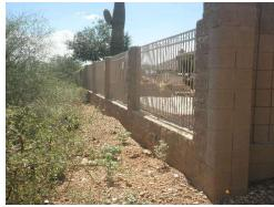
Fair to good condition. Rust visible in some locations. Includes: (4) entry/exit gates, (3) pedestrian gates, fencing along south perimeter next to lot 32, fencing at the ends of cul-desacs on west perimeter and view fencing along boundry lines between lots and common areas. Approximately 7,760 LF of fencing. Last painted by Advanced Painting & Contracting in 3/16 for \$38,304. Cost savings due to masonry walls and metal painting in same year.
