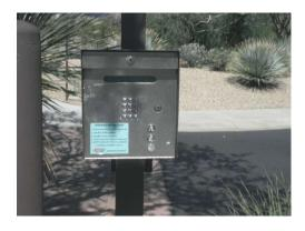
Located at 128th Street and Via Linda entry gates. Door King entry access phones. Interior board equipment replaced in 2017 for \$1800 & \$1400 each.
