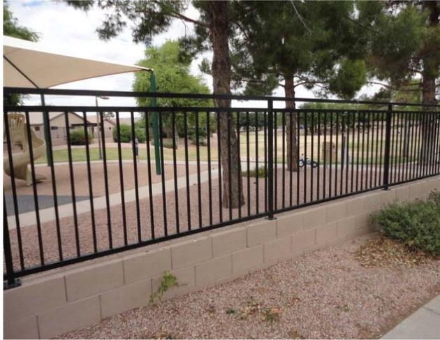
The client has advised us that \$40,527 was spent in June 2016 to repair & repaint the wrought iron fencing throughout the community. This component budgets to repair & repaint the wrought iron fencing every five (5) years, and includes a provision to repaint the steel split rail fencing.
