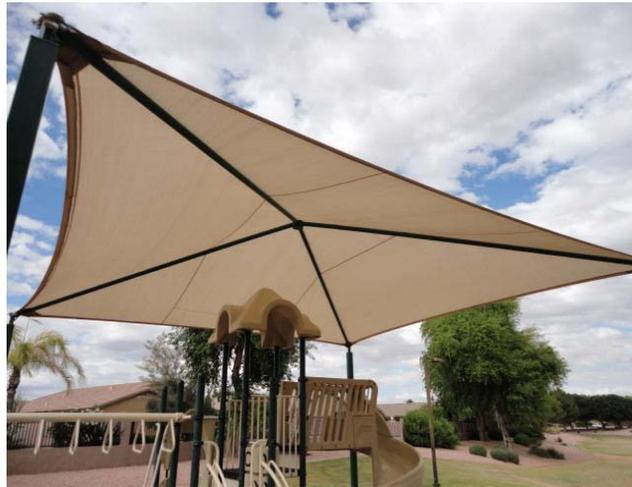
This component budgets to replace the shade structure fabric (hip/ridge) in conjunction with the replacement of the playstructure.
