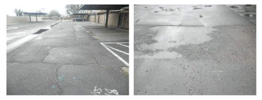
Poor to Fair condition. Recommend sullry seal to extend the life of the pavement. Should include crack sealing prior to slurry seal. One time application.
