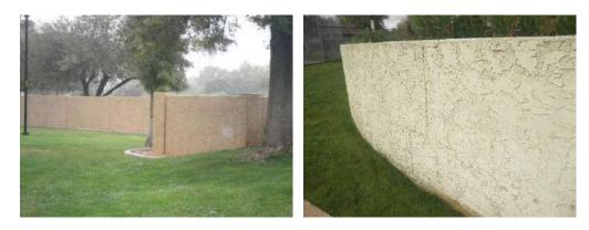
Good to fair condition. Some cracking and poor paint on interior walls at pool recreation area. Outside walls in surrounding community good condition. Last repaint date unknown.
