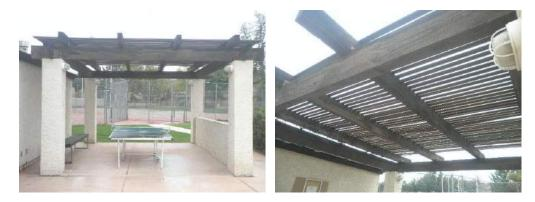
Good condition. Stucco posts with wood supports and metal slats. Ramada next to pool equipment building in pool recreation area. Estimate wood structure to last another 5 years so long as upkeep is maintained. Noted wood deteriorating from sun and weather exposure.
