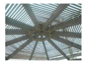
Good condition. Stucco posts with wood supports and metal slats. Ramada location is covering spa in pool recreation area. Estimate wood structure to last another 5 years so long as upkeep is maintained. Noted wood deteriorating from sun and weather exposure.
