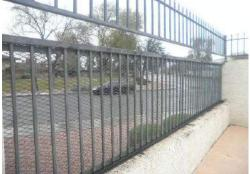
Poor condition. Surrounding pool recreation area. Rust and detrioration evidient where spray irrigation hits. Last repaint date unknown.
