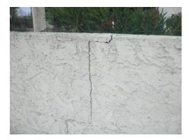
Good to fair condition. Some cracked and poor paint on interior walls at pool recreation area. Outside walls in surrounding community good condition. A budget for making wall repairs on a 5 year recurring schedule with approximate replacement of 1%. Total of approximately 20000 sf.
