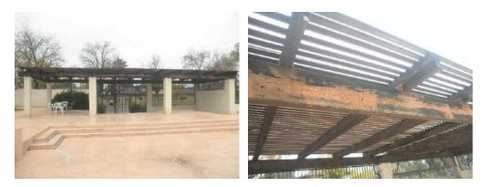
Good condition. Stucco posts with wood supports and metal slats. Ramada is at entrance to pool recreation area. Estimate wood structure to last another 5 years so long as upkeep is maintained. Noted wood deteriorating from sun and weather exposure.
