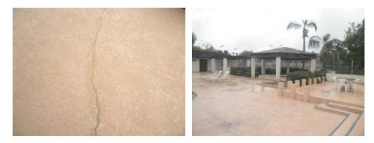
Good to fair condition. Some limited cracking. Suggest cleaning. Date of last recoat unknown.
