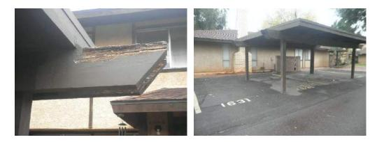
Good condition except where wood exposed (showing dry rot) on ends protruding from Asphalt roofs.
