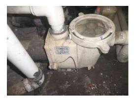
Poor condition. Whisperflow 3/4 hp. Leaking. Suggest replacing along with spa motor. Last replacement unknown.
