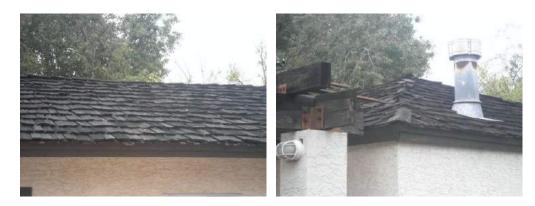
Poor condition. No signs of leaking but noticable movement away from roof. Our cost is based on replacing with a composite 20 year shingle.
