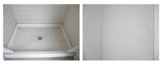
Good condition. Needs cleaning and paint. Ceramic tile floor to ceiling above pan.
