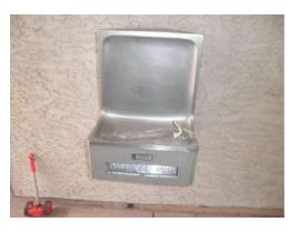
Non usable condition. Broken and disconnected. Elkay.
