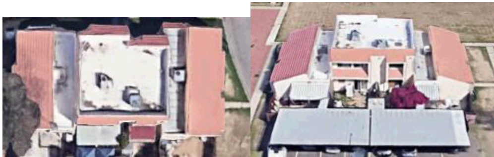
Roofing Southwest replaced in 2018.
