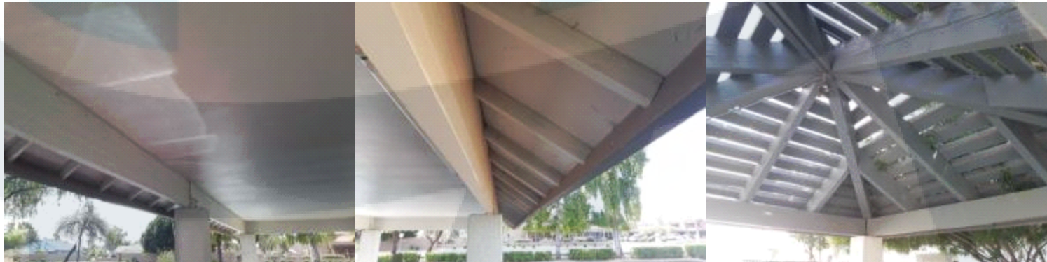
Funding to repaint wood ramada at pool, carport's trim and ceiling.
