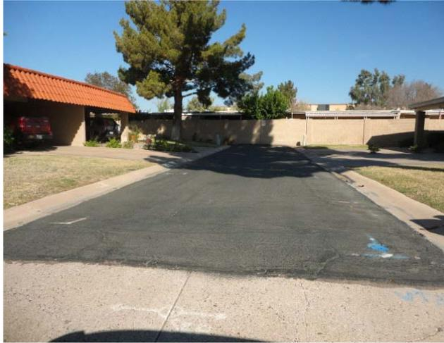
This component budgets for a continuous four (4) year seal coating cycle beginning in 2022, six months after the new asphalt is installed.
