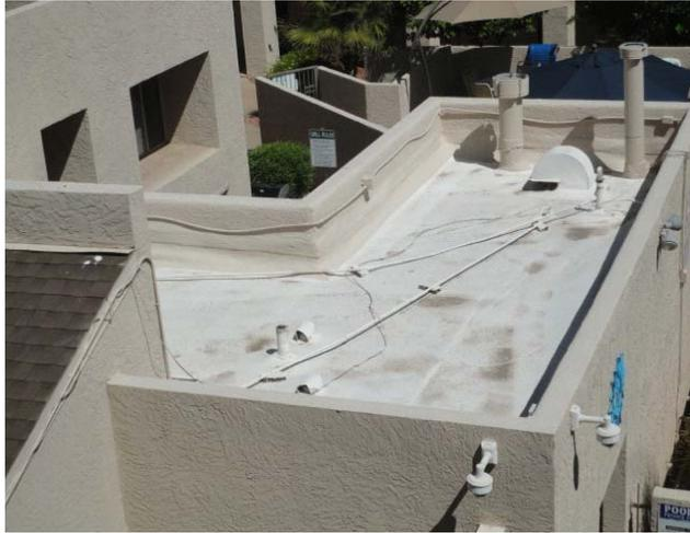
This component budgets for an elastomeric recoat of the flat, foam roofs atop the four (4) residential buildings, the storage building and the clubhouse on a 10 year cycle. It appears that Progressive Services completed a project in late 2015 for \$98,895 to replace the foam roofs or complete major repairs and recoat. We have used 1/2016 as the basis for aging these roofs and have scheduled the next recoat for 2026.
