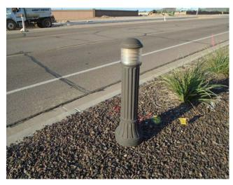
There are 89, 3'6" metal bollard light fixtures scattered throughout the community. In late 2016/early 2017, \$21,280 was spent to install 76 new LED retro lighting systems to change the existing ballast and lamp bollards to LED HPS (soft white) or LED Metal Halied (bright white). We have assumed that the other 13 bollards were done previously, or done after (no information on the other 13 bollards was provided).
