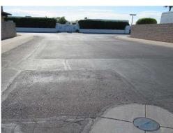
Per Holbrook Asphalt's 30 year plan, this component is for application of a armor coat in 2022 and 2043 following slurry seal applications.
