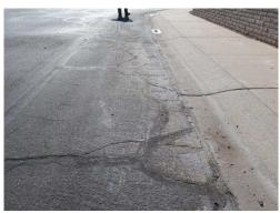
Poor to fair condition. Approximately 78,025 sf. Per Holbrook Asphalt's 30 year plan slurry seal is recommended in 2021 and 2042.
