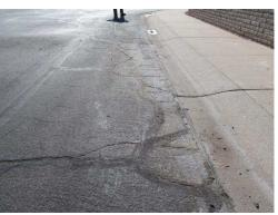
Poor to fair condition. Approximately 78,025 sf. Per Holbrook Asphalt's 30 year plan slurry
