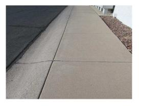
Good condition. Noted some minimal cracking and some repair work performed. Includes sidewalks and curbing. This component provides a budget for concrete repairs on a 5 year recurring cycle.
