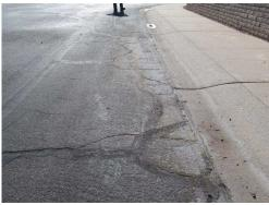
Poor to fair condition. Approximately 78,025 sf. Per Holbrook Asphalt's 30 year plan, patching/repair is budgeted for 2031, 2041 and 2051.
