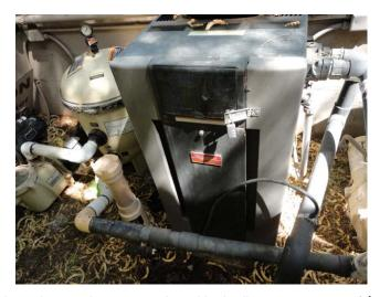
This is a Raypak, 206,000 BTU input heater that was replaced in April 2014 at a cost of \$2,374.76.
