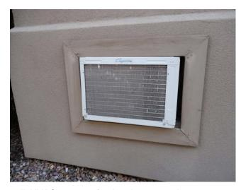
These are Comfort Aire, thru-the-wall, HVAC systems for the elevator equipment rooms at Buildings 5, 6, & 8.
