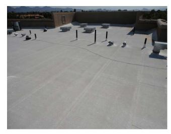
The flat, built-up roofs atop the four condominium buildings received an elastomeric coating in 2011/2012. This component budgets to replace the flat, built-up roofs atop the condominium buildings on a 20 year cycle. Accumulated funds can be used to recoat these roofs if desired by the client. Should this occur, the useful life cycle of these roofs can be reevaluated.
