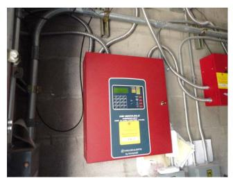
The Building 7 fire alarm control panel (Fire Lite, MS-9200UDLS) was replaced in February 2013 at a cost of \$1,792.23. The fire alarm control panel (Fire Lite, MS-9200UDLS) at Building 8 appears to have been replaced around the same time. For budgeting purposes we have used 2014 as an average placed in service date for these two fire alarm control panels.
