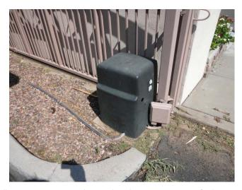
These are Elite, SL-3000-UL sliding gate operators located at the east entrance/exit gates.
