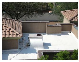
The flat roofs atop the four townhome buildings appear to have all been foamed between 2015 & 2017. For budgeting purposes we have used 2016 as an average placed in service date for these roofs. This component budgets to repair & recoat the foam roofs on a continuous 10 year cycle.
