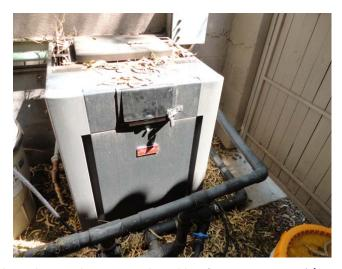
This is a Raypak, 400,000 BTU input heater that was replaced in 1/2014 at a cost of \$2,989.99.
