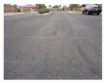
The asphalt was crack sealed & seal coated in October 2014 at a cost of \$17,445.82. This component budgets for similar work every four (4) years.
