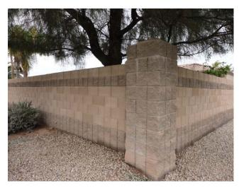
There is approximately 38,000 sq. ft. of perimeter & interior common area facing block walls. In late 2016, \$5,856 was spent to replace two sections of walls. Going forward, this component will accumulate funds on a 10 year cycle for block wall repairs/replacements on an "as needed" basis. The budgeted amount and useful life cycle should be adjusted over time as wall conditions dictate.
