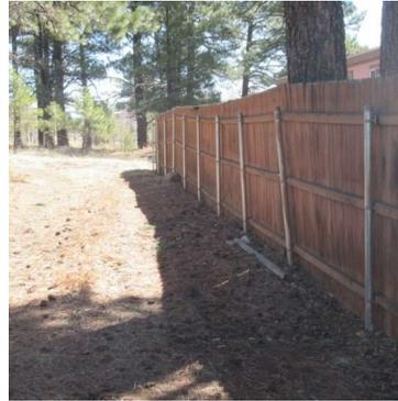
Faded condition. Approximately 3,200 ft of fence. Condition of fence stain varies. Budget based on staining in 2023.
