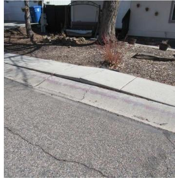
This asset is for \$2,500 every 5 years to be used "as needed" to repair concrete components including but not limited to: basketball court (approximately 35' x 50'), concrete drainage swales, sidewalks, etc. Noted some repairs to swales along with cracks, dips and lifted areas on sidewalks.
