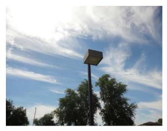
These are pole mounted, box style fixtures at the three (3) basketball courts. The cost does not include the replacement of poles or mounting brackets.
