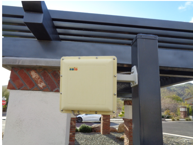
This is an Applied Wireless ID, LR-3000 RFID reader.
