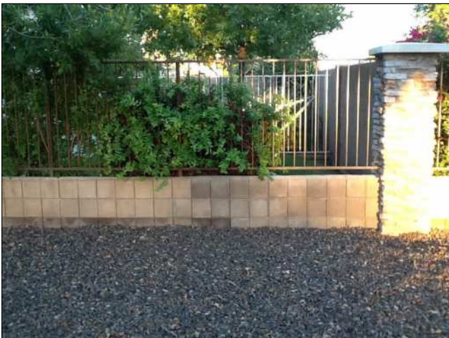
Paint CMU Wall and Wrought Iron Fence
