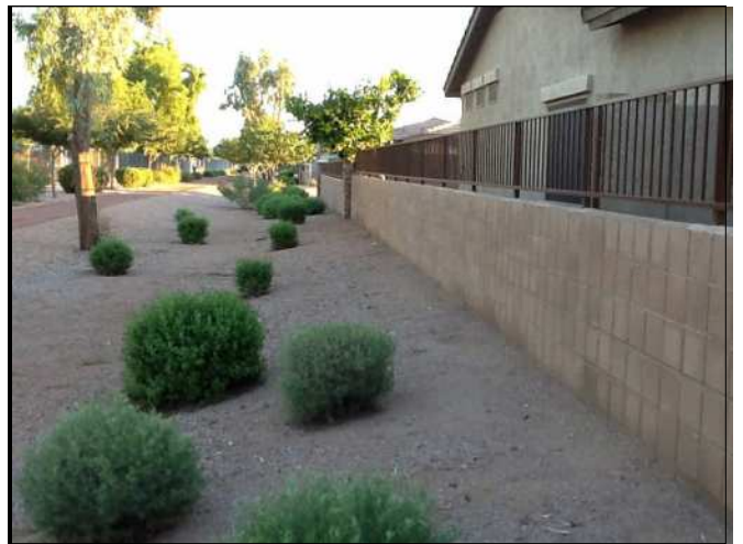
Paint CMU Wall and Wrought Iron Fence
