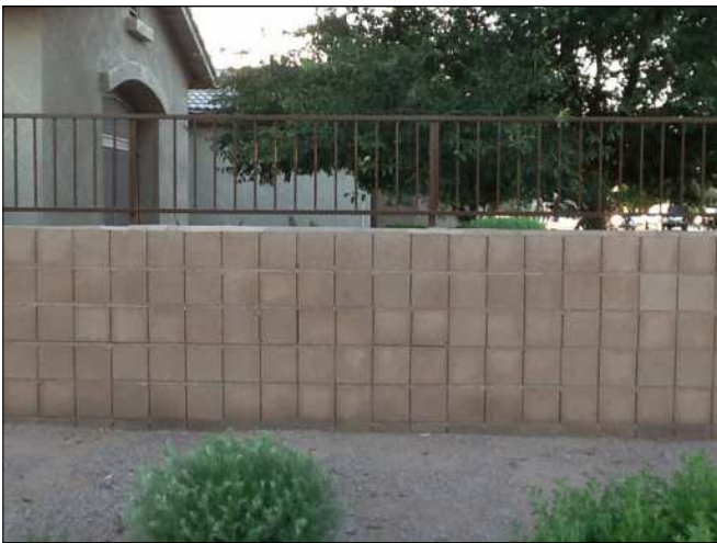
Paint CMU Wall and Wrought Iron Fence
