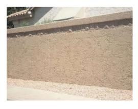
Good condition. This asset includes repair and painting of stucco masonry walls. Approximately 109,000 SF of community walls. Walls painted in 2018 for a total of \$106,849.98.
