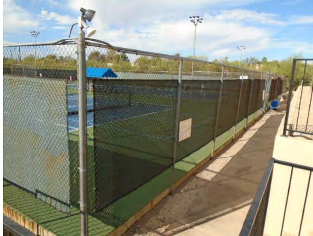
The 9' chain link fencing & gates appear to be original from 1978. We are budgeting to replace this chain link in 2030, and then on a 40 year cycle.
