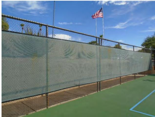
This component budgets to replace the 335 LF of 6'3" high windscreens attached to the chain link fencing at the tennis courts.
