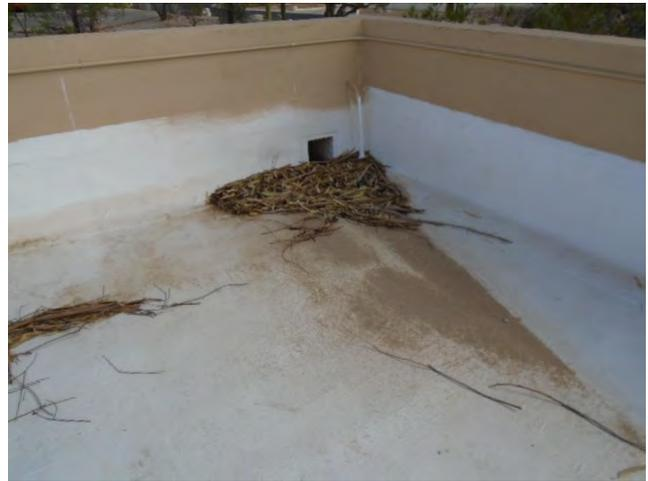
The flat, built-up roofs atop the clubhouse & pool area ramada were coated/recoated in mid-2022. This component budgets to coat/recoat these roofs on a five (5) year cycle.
