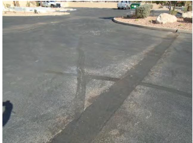
The parking lot asphalt was crack sealed, seal coated & restriped in mid-2022 by Bates Paving & Sealing, Inc. at a cost of \$6,527. This component budgets for similar work every five (5) years, and also includes a provision for asphalt repairs.
