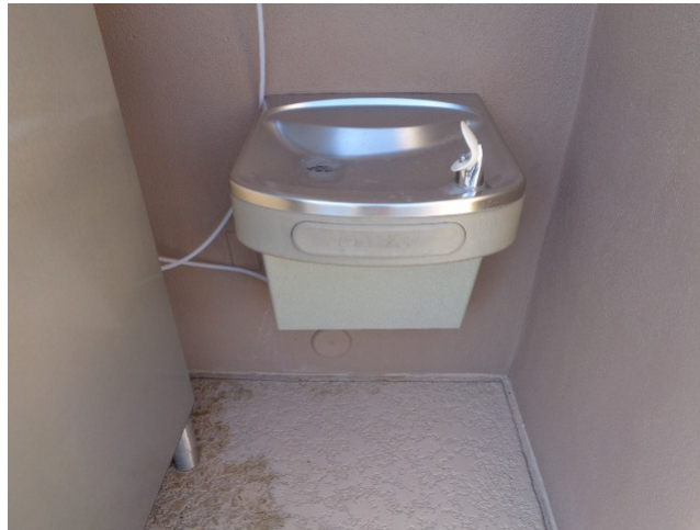
This Elkay drinking fountain is wall mounted to the Great Room building.
