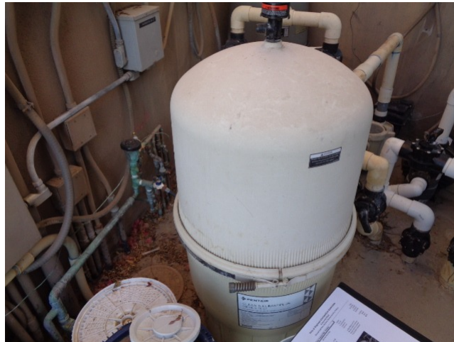
This is a Pentair, Clean & Clear Plus, 420 sq. ft. cartridge filter.
