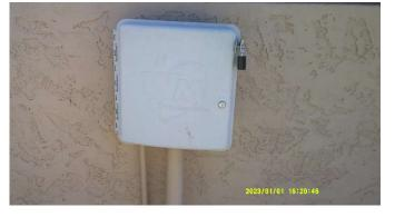
(1) 36 station Weathermatic SL4800 Smart Timers irrigation controller @ Saddle Park & (1) 24 station Weathermatic SL4800 Smart Timers irrigation controller @ Abilene Park. There are many more smaller controllers located throughout the community - see asset ID 1022.
