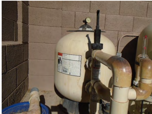
The Triton II, 3.14 sq. ft. sand filter (manufactured 1/12/2015).
