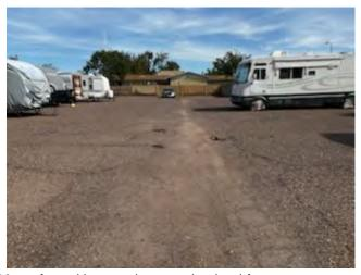
The RV Lot asphalt measures 14,700 sq. ft. and has not been maintained for many years and has not been budgeted for maintenance in the reserve study for some time. It is in poor condition but is serving its purpose and will continue to do so, even when it deteriorates to the point of being dirt. That being said, if the Board would like us to include budgeting to remove and repave or chip seal this lot, we will do so upon request in a revision or future updaate of this report.
