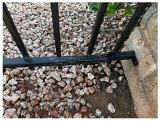
The pool wrought iron is in varying condition based on whether it is hit by spinkler water or not. There is some base rail rusting but overall is in fair condition. Some base rail repairs may be needed using funds from the annual operating budget. We have scheduled full replacement for 2035.
