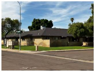
This component budgets to replace the asphalt shingle roofs atop the condominiums buildings. \$615,000 was spent in 6/2006 to remove and replace the wood shake roofs with 30-year laminated fiberglass shingles (cost also included new 1/2" OSB, 2" galvanized metal drip edges around the perimeter of the roofs and two (2) layers of 30# felt underlayment.
