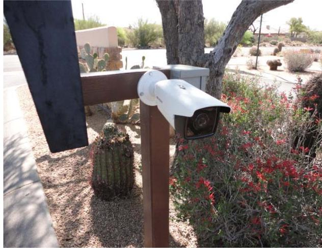
There are four cameras at the Dusty Coyote Circle entrance/exit area. We have assumed that there is also a DVR located somewhere. We have estimated that these components were installed in 2017 (no information was provided by the client). This component includes a provision to replace the surveillance components every seven years.
